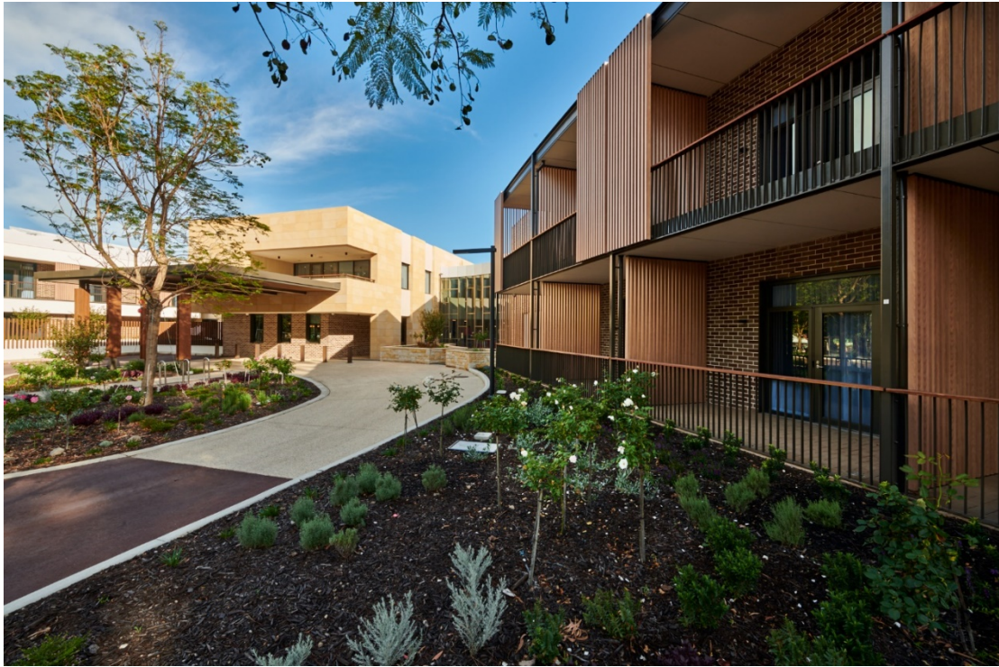
Karingal Green - Front facade
